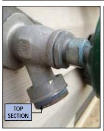
IMPORTANT: After installation, vacuum breaker may need to be pressurized to work correctly: hook up a hose with a closed nozzle attached, turn the faucet on FULL BLAST and allow hose to fill. Once filled, the vacuum breaker will seal & stop leaking
