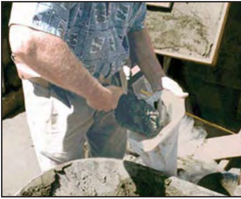
1. Fill grout bag using a trowel.
