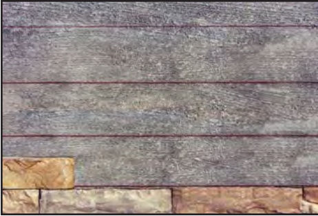
Applying First course of stone
