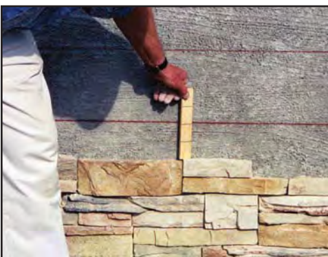
Using a measuring stick
