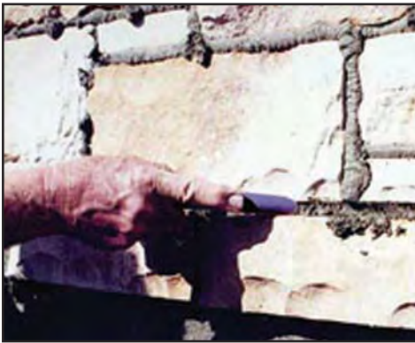
4. Using the back of a wire brush, stick or something similar, press the mortar into the joints as the mortar is beginning to set and before it gets too hard. When this process is done too soon the mortar can smear on the face of the stone or give the grout a slick look.
