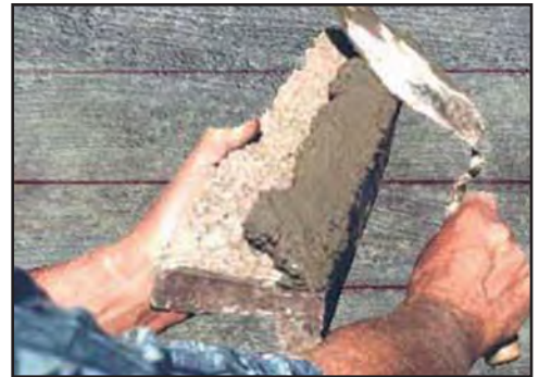
Applying mortar to stone
