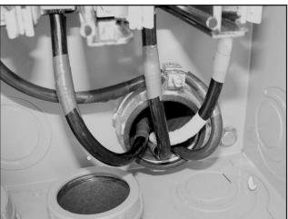
k) Raceway terminations shall be made up tight. Where terminations are subject to vibration, bonding bushings or wedges shall be used to assure electrical continuity. Where subject to vibration or dampness, insulating bushings shall be used to protect the conductors (see Figure 9).
