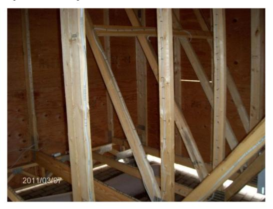
Figure 19 - NM cables installed on wood studs
