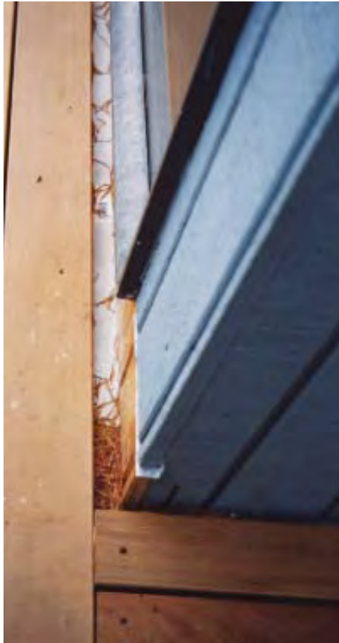
Figure 4. Although it's common practice to bring an L-shaped flashing down the wall and kick it out over the ledger, the resulting pocket can collect debris, and rot both the decking and the siding above.
