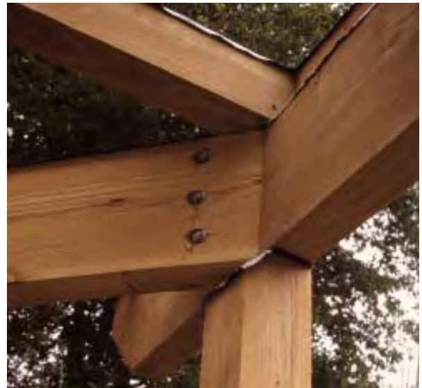
Figure 9. To keep this deck – which is framed with untreated lumber – from rotting, the author coated it with a borate preservative and covered the upper surfaces with torch-down roofing membrane.
