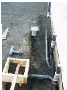
Shower access box in concrete floor.
