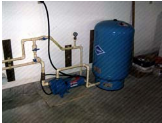
.Water pressure can be increased with a well pump and bellows tank.
