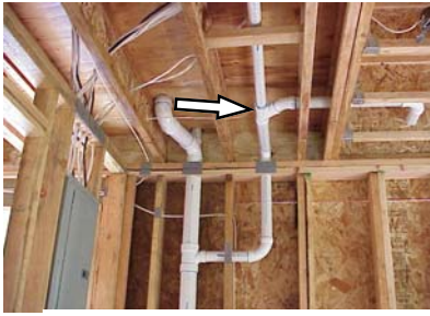
Combination y-1/8 bend in horizontal position.
