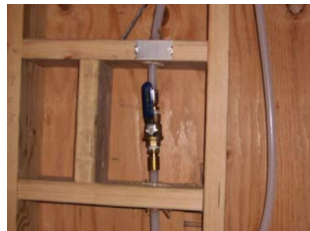
Connection of valve in wall. Wall framed for valve access.
