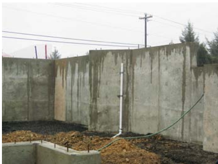
Ten foot head of water for test of under slab plumbing.
