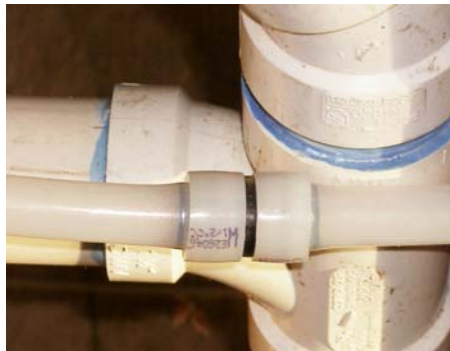
Wirsbo Pex coupling with memory ring. Use inside house or outside in ground.
