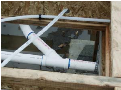
Connecting horizontal drain to horizontal drain with Y fitting.
