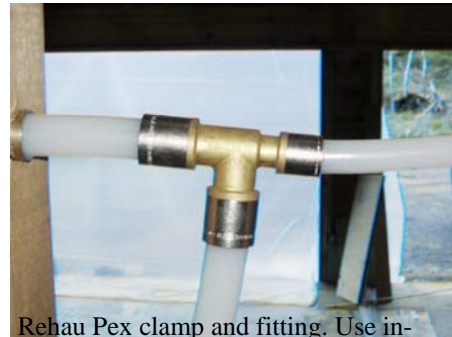
Rehau Pex clamp and fitting. Use inside house or outside in ground.
