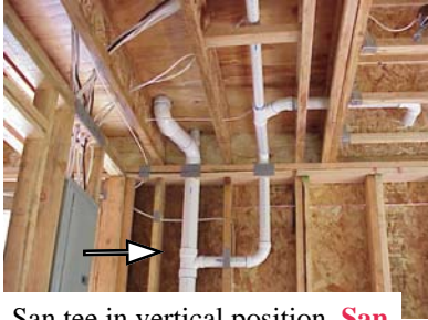
San tee in vertical position. San tee in horizontal position not permitted as drainage fitting.
