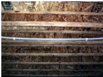
Strap water pipe using chart above.
