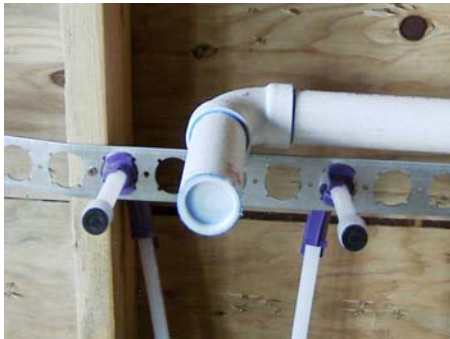
Cap all waste and water lines for test.
