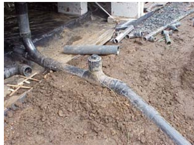
Two way cleanout tee .To be used just outside of the building foundation on the sewer drain line.
