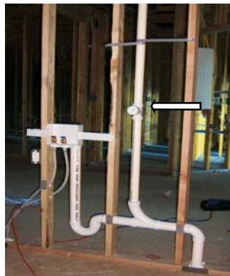
Cleanout above washer so it can be used without moving washer
