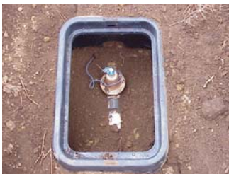
With water pressure over 80 psi a pressure regulator is required.
