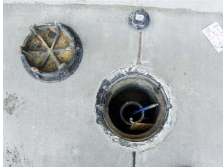
Test plug in cleanout. Filled with 30 Lb. Air.
