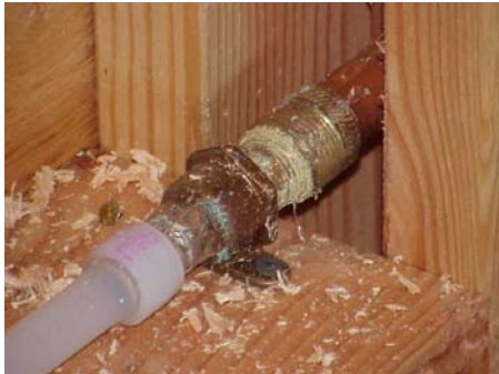
Wirsbo Pex water pipe fastened to structure for hose bib outside.
