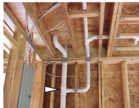
Waste connection downstream of toilet
