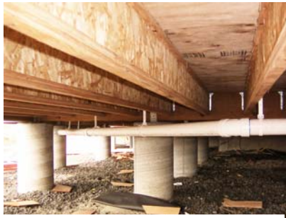
Hang ABS or PVC waste pipe at 4 foot on center.
