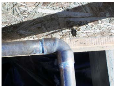
Copper pipe and fitting. Soldered with lead free solder. Use inside house or outside in ground.
