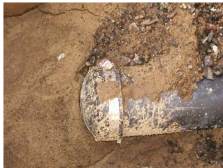
Test cap on sewer line.
