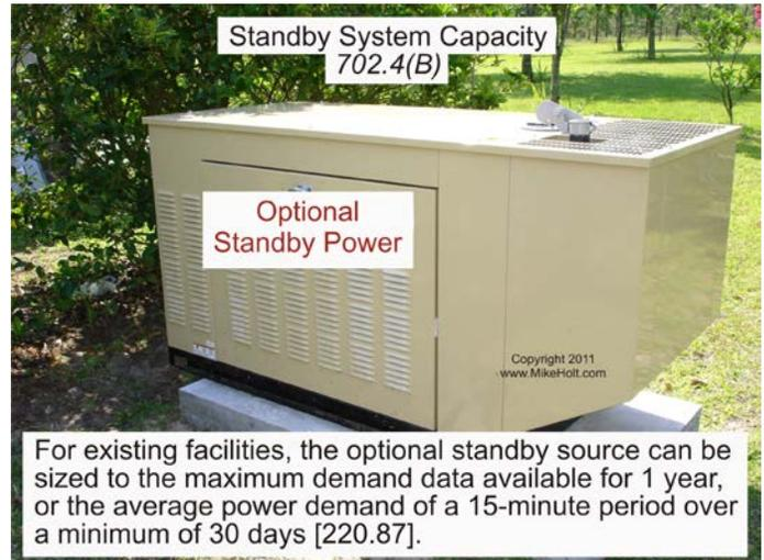
For existing facilities, the optional standby source can be sized to the maximum demand data available for 1 year, or the average power demand of a 15-minute period over a minimum of 30 days [220.87].
