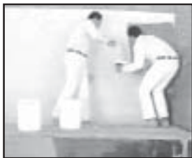
Applying the Finish
