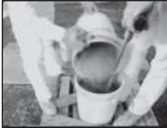
Mixing the Adhesive - A 2-Man Job
