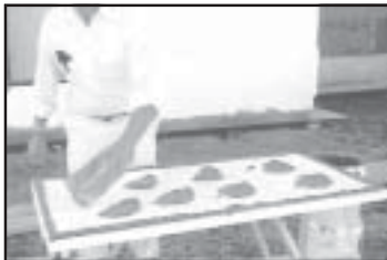
Applying the Adhesive
