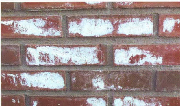
Figure 1. Typical white efflorescent salts on brick and block masonry
