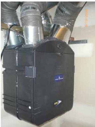
*This is one example of a heat recovery ventilator located within a conditioned space. Source: O'Brien & Company.*
