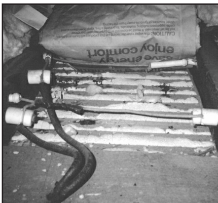
Figure 5 - Paper Faced Insulation
