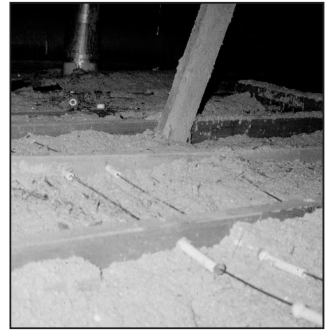
Figure 7 — Non-Flammable Insulation
