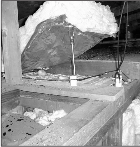
Figure 6 — Foil-Faced Insulation
