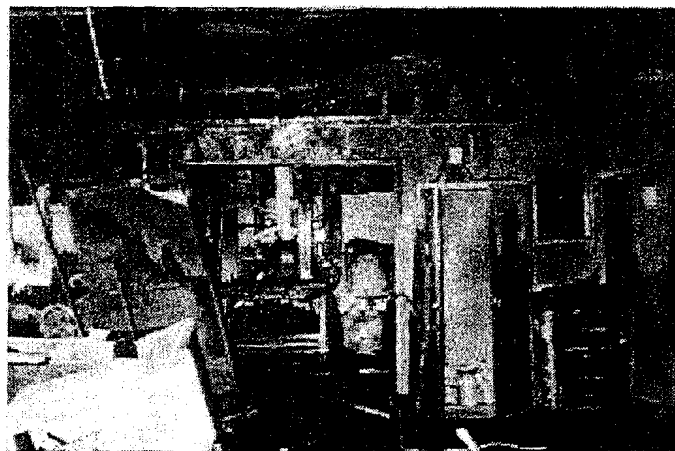
Figure 4.3. —Area of fire origin in Building 2 fire at the Forest Products Laboratory,
