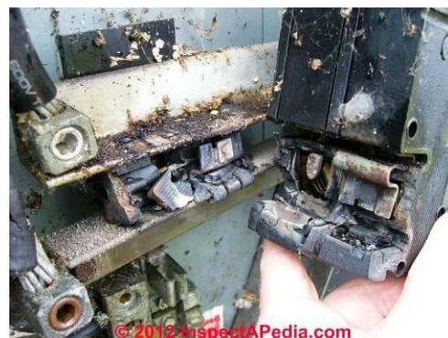
**Fig. 10. Burned Zinsco™ Main Circuit Breaker and Burned Zinsco™ Electrical Panel Bus.**
