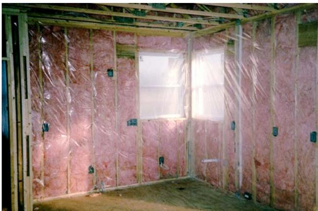
**Photograph 1: Plastic Vapor Barrier**—Not a “production friendly” method of achieving airtightness and it was not “robust” in terms of surviving the construction process and in providing performance over the service life of the building. It was also climate sensitive. It made no sense for assemblies that saw air conditioning – it was a vapor barrier on the wrong side of such assemblies.
