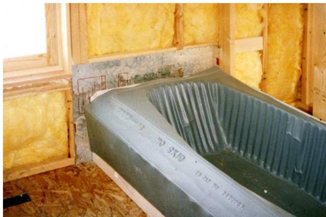
**Photograph 3: Bathtub on Exterior Wall**—Targeting the big holes with rigid draft-stopping. Of course an even better approach is not have a bathtub on an exterior wall...
