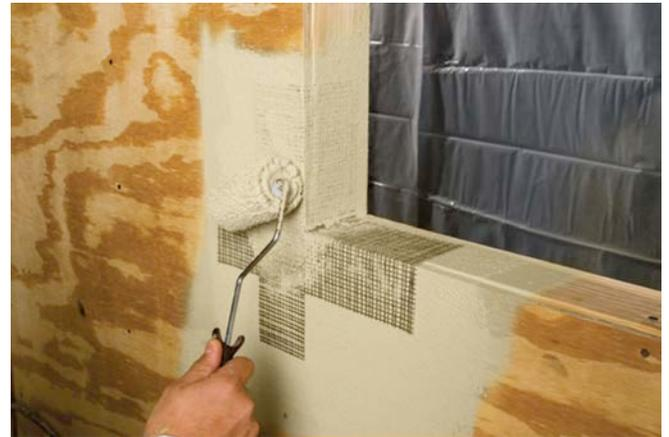
**Photograph 12: Another Window Opening—**Some systems require fabric reinforcement at critical interfaces.
