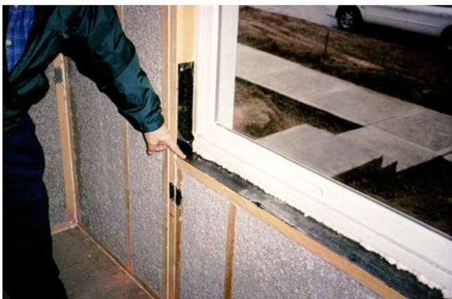
**Photograph 2: Interior Gypsum Board as the Air Barrier**—Note the sealant at the bottom plates an around window openings.
